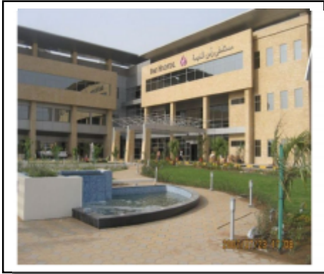
G +2 Story Hospital Bldg/R.A.K
