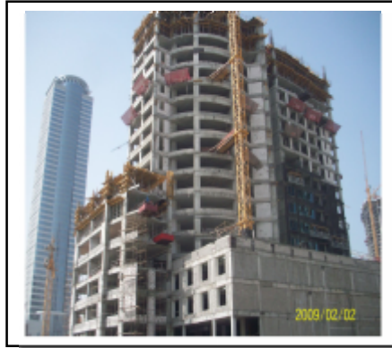
Ontario Tower–Business Bay–Dubai
